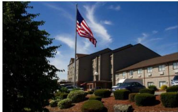
Earlier this year, Thorofare Capital provided a $17.75 million bridge loan to a New York real estate developer for the acquisition, renovation and rebranding of a 200-room Mainstay Hotel in Newport, Rhode Island. The non-recourse financing included a 33-month term and interest-only payments.
